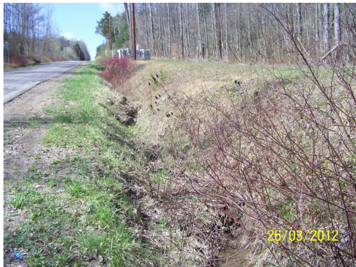
Photo 1: Bly Hill pre-ditch stabilization
