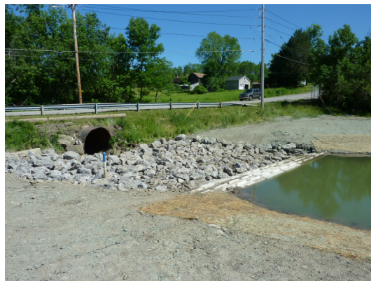
Photo 7: Post installation of debris basin and constructed wetland
