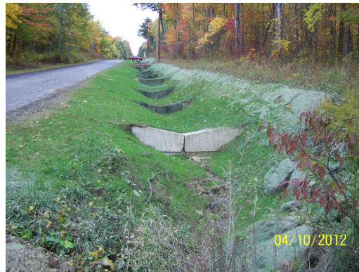
Photo 2: Bly Hill post-ditch stabilization
