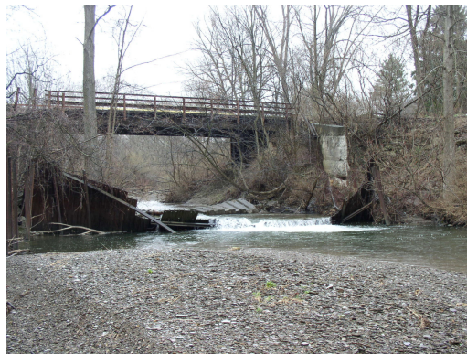
Photo 8: Pre- weir and grade stabilization
