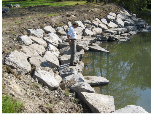
Photo 6: Post streambank stabilization
