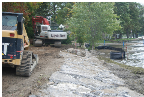
Photo 10: Post shoreline stabilization
