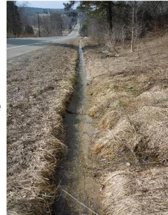
Drainage Ditch Along Route 430
