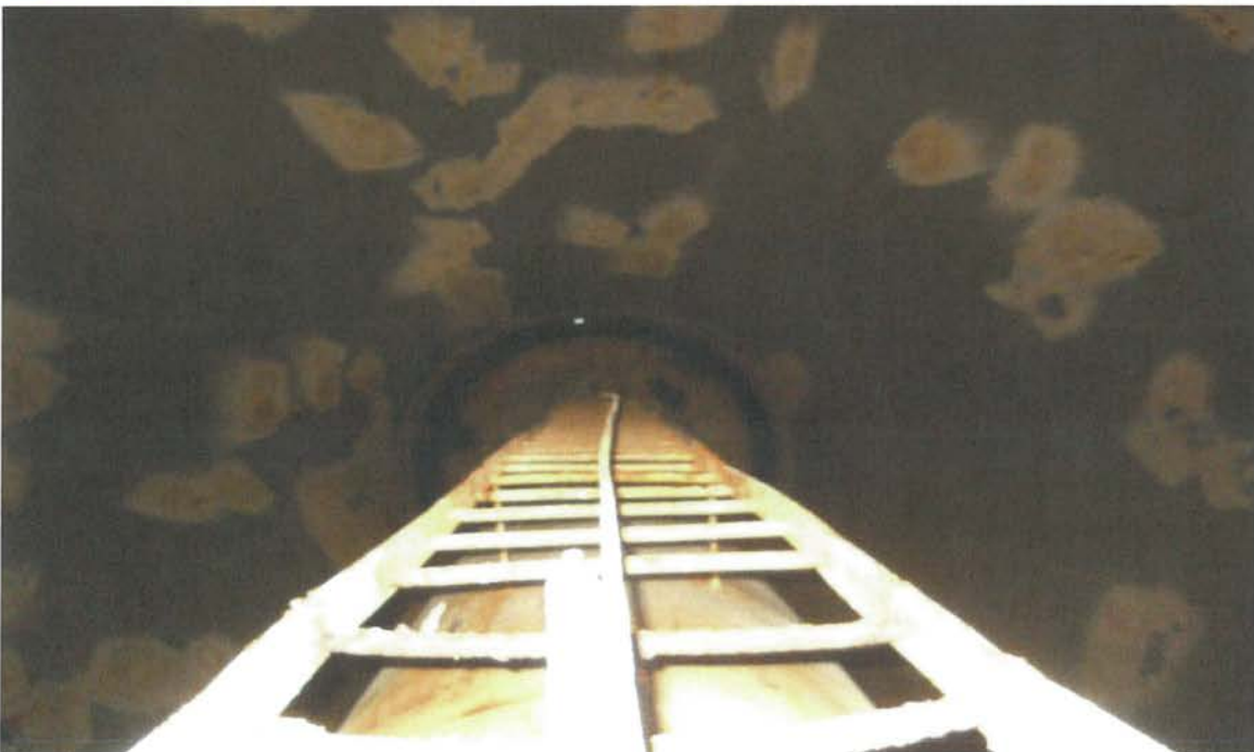
Photos show the tank interior during the cleanout process.
